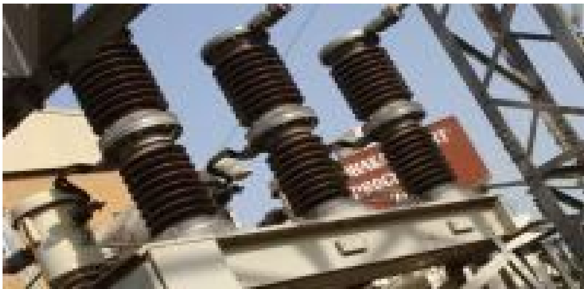
Figure 7: DCS (Containing AVR, CT, PT) (author)
