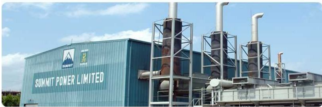
Figure 4: Summit Power Plant, Ashulia [2]
