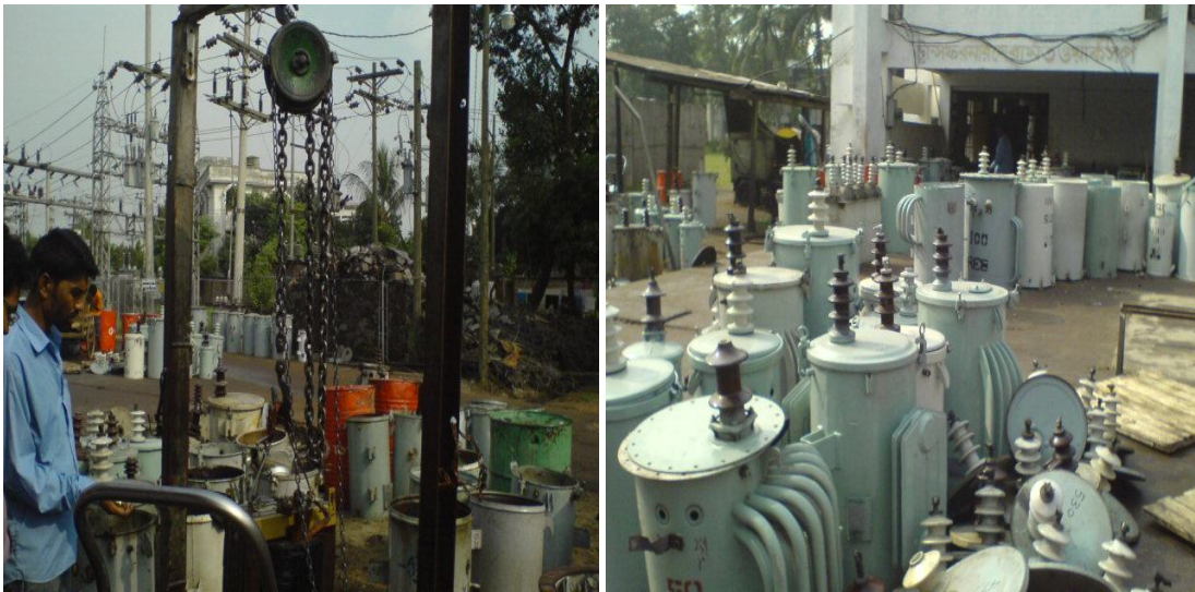
Figure 21: Repairing Transformer at PBS-1 (author)
