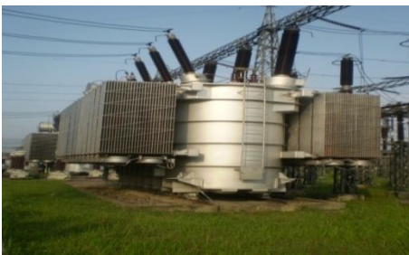
Figure 4.4: Intermediate Transformer
