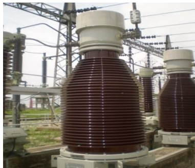
Figure 4.3: Current Transformer
