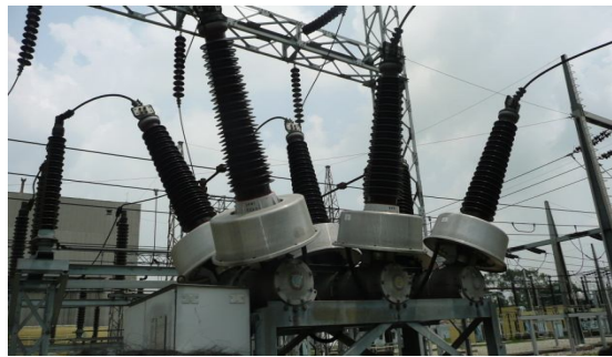
Figure 4.11: SF6 Circuit Breaker
