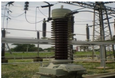
Figure 4.4: Potential Transformer
