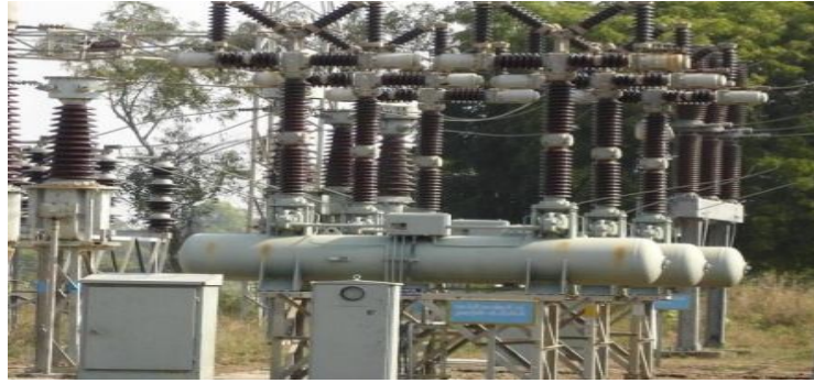
Figure 4.12: Air blast circuit Breaker
