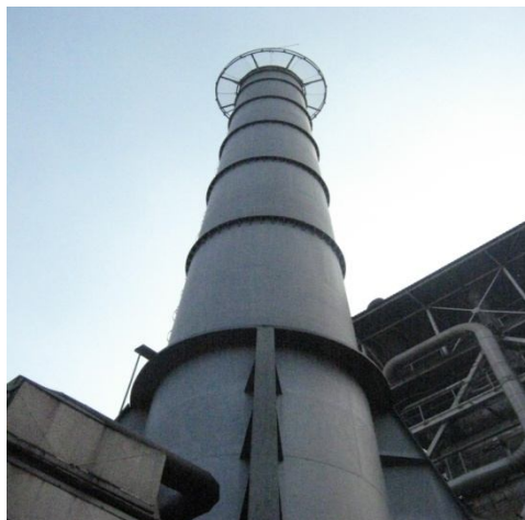
Figure 2.10: Stack/Chimney of unit-2
