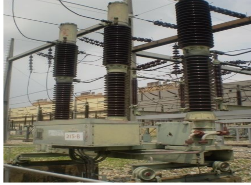
Figure 4.10: Oil Circuit Breaker
