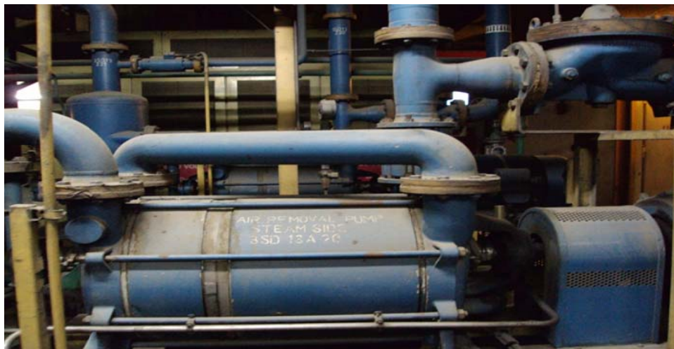
Figure 3.10: Air removal pump
