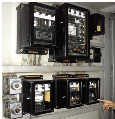
Figure 6.9: Different types of relay used at APSCL
