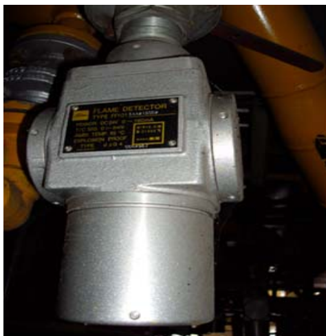
Figure 5.4: Flame detector
