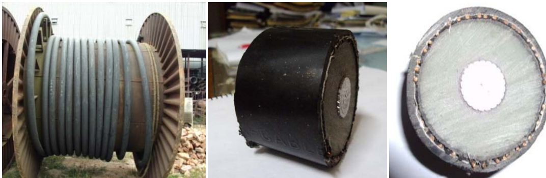
Figure 6.23: XLPE insulated Underground Power Cable used in APSCL
