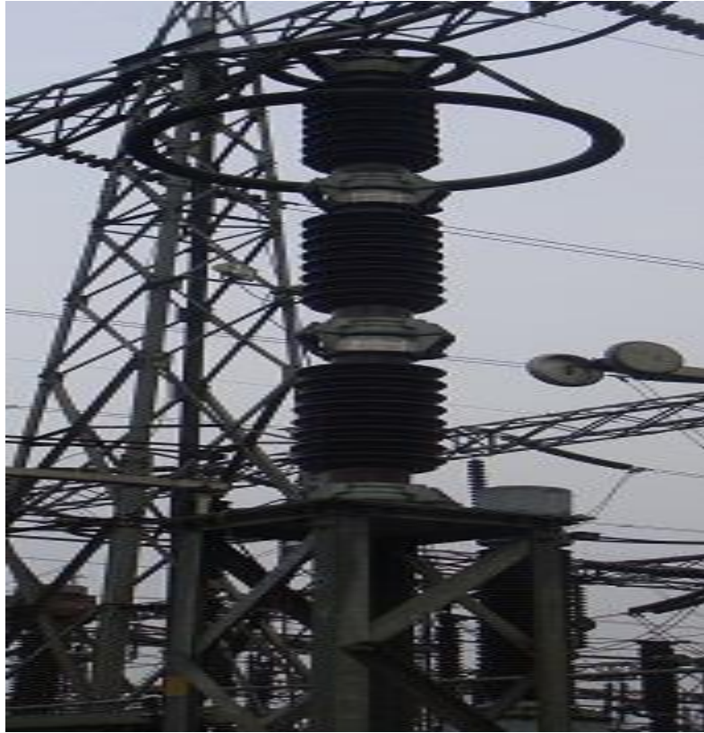
Figure 4.8: Lightning Arrester. [Source: Author]
