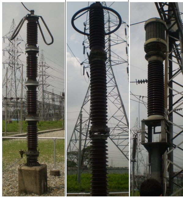
Figure 5.3: Various Types of Lighting Arrester [7].
