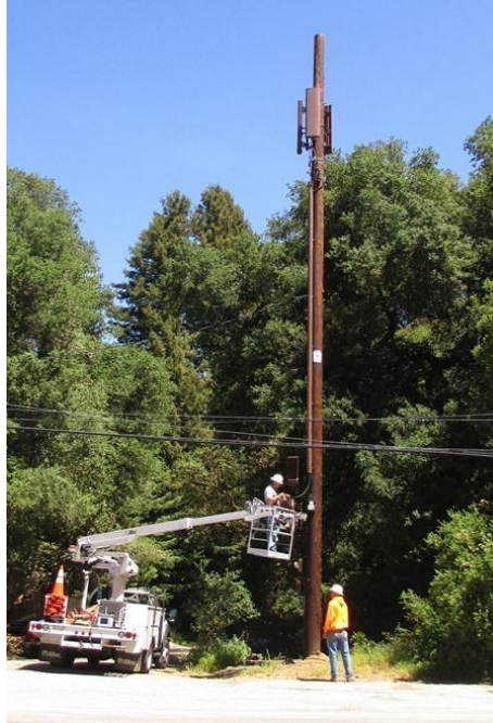
Figure 5.2 Bucket truck in use at quasi-Omni, small cell installation
