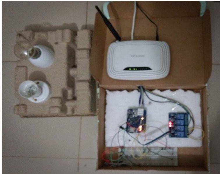
Figure 5.2: Connection with load when device in OFF mode
