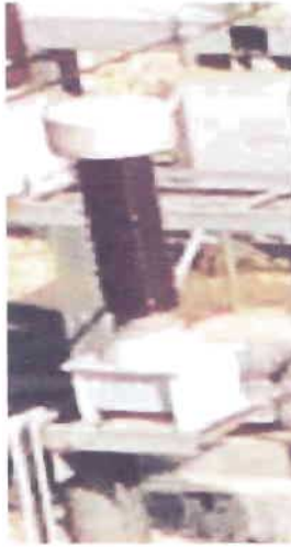
Figure 3.6: 145 kV single phase outdoor types Potential Transformer by ABB (Sweden)
