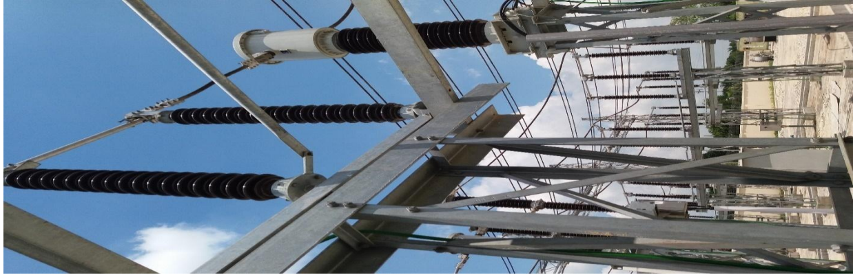
Fig 5.3: SF 6 circuit breaker
