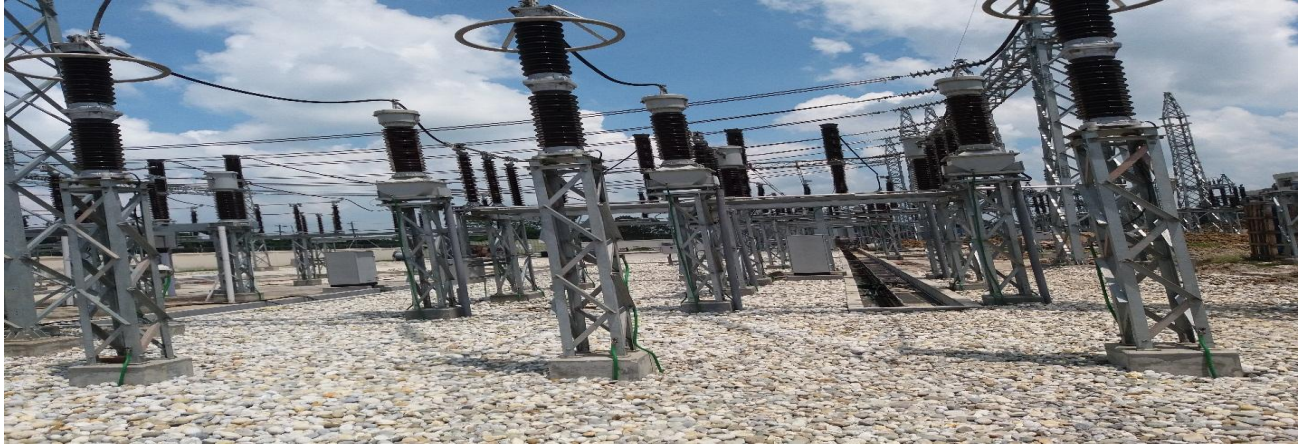
Fig 5.5: Lightning Arrester
