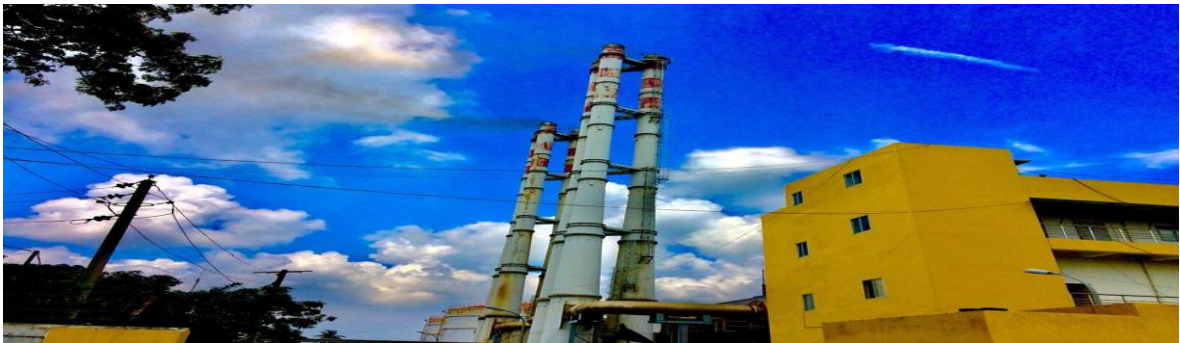
Fig 2.7: Chimney of Katakali peaking power plant
