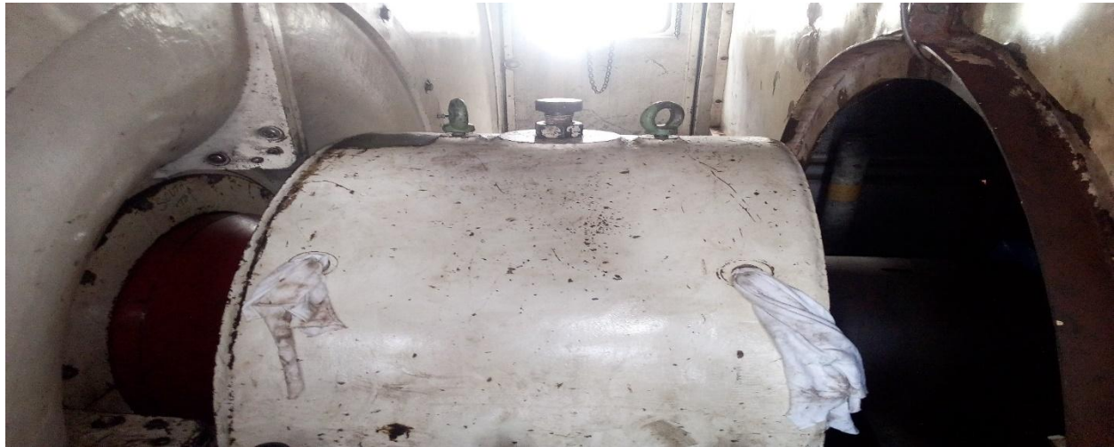
Fig 3.5: Turbine and combustion chamber is coupled through a Shaft
