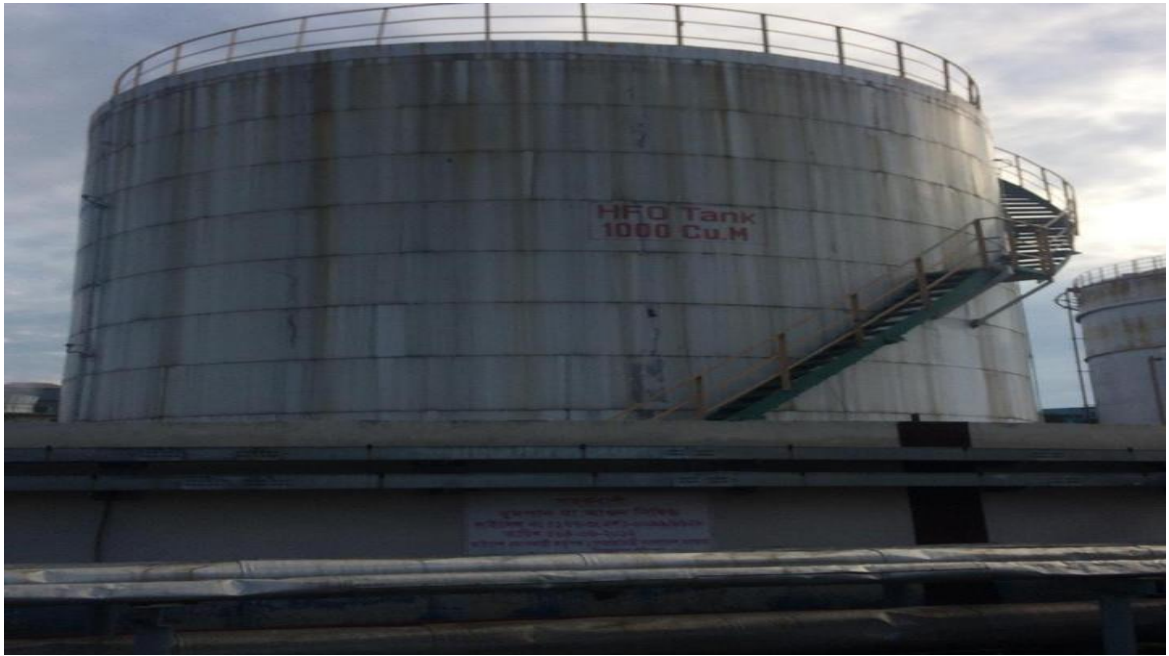
Fig 2.1: HFO tank at Katakali peaking power plant
